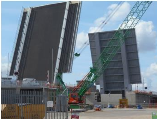
The new Herring Bridge
